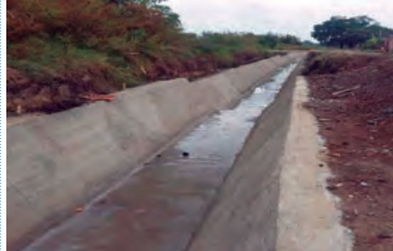
Construction of water canal for risk mitigation at Suerte Cuarenta Neighborhood.
