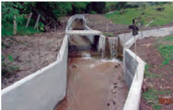
Canalization of Borrigueros creek.
